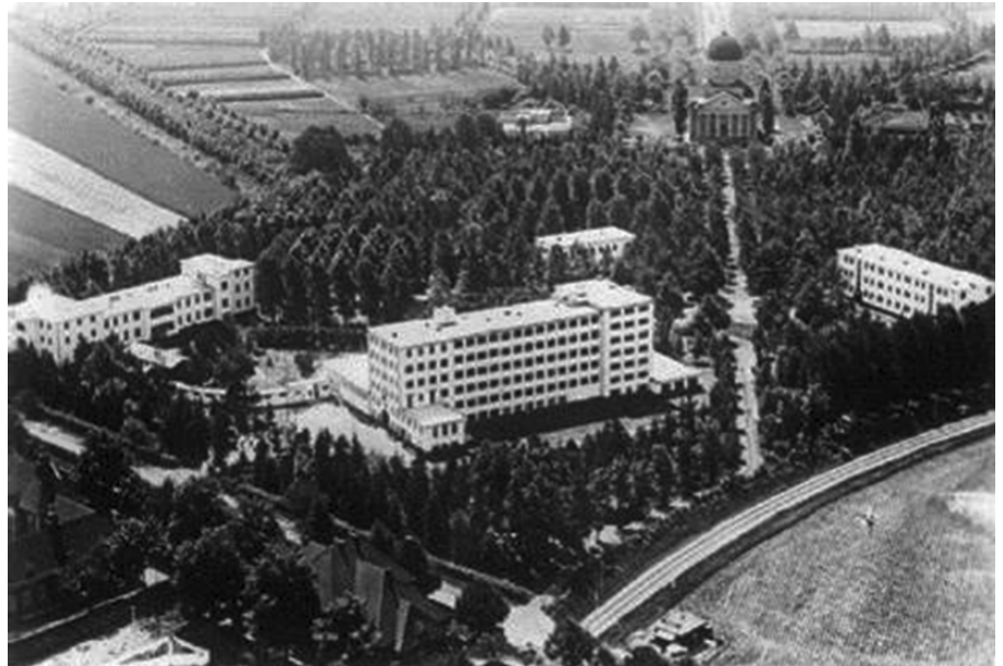
Fig. 4. Building of the KWI for Brain Research in Berlin-Buch (1931; from [26], with permission of Springer-Verlag).
